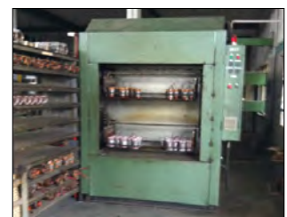
Stator Varnish Plant
